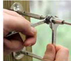
Step 2 Tighten cone onto receiver.
