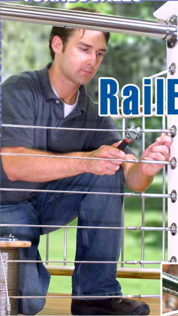
Step 1 Fully seat wire rope.
