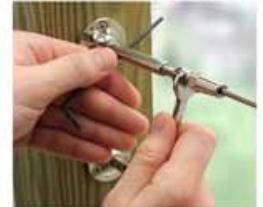
Step 3 Rotate body to tension wire rope.
