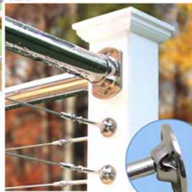
Step 1 Fully seat wire rope.
